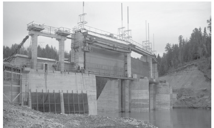
Bearspaw Dam under construction, 1954 (Glenbow Library and Archives Collection)
