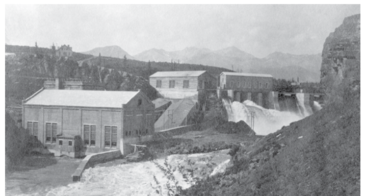
Horseshoe Falls dam and power plant, 1913 (Glenbow Library and Archives Collection)
