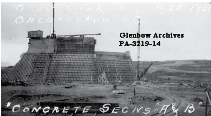
Construction of Ghost River dam, ca. 1928-1930 (Glenbow Library and Archives Collection)
