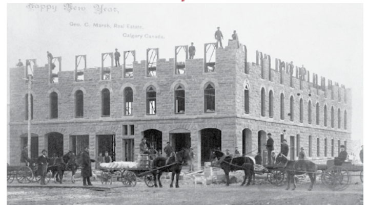
Alberta Hotel under construction, Calgary, Alberta., 1888-12-20, (CU1127189) by Ross, Alexander J. Courtesy of Libraries and Cultural Resources Digital Collections, University of Calgary.
