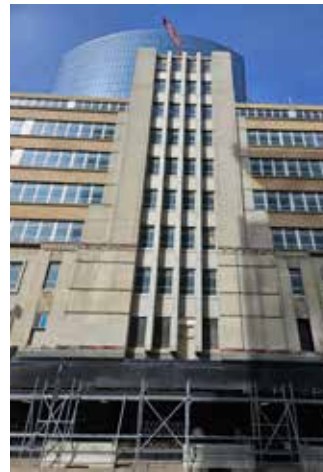
Barron Building undergoing renovations, 2023 (Anthony Imbrogno)
