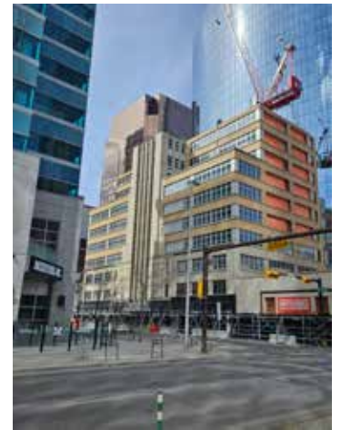
Barron Building undergoing renovations, 2023 (Anthony Imbrogno)
