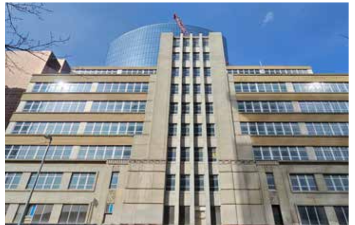
Barron Building undergoing renovations, 2023 (Anthony Imbrogno)
